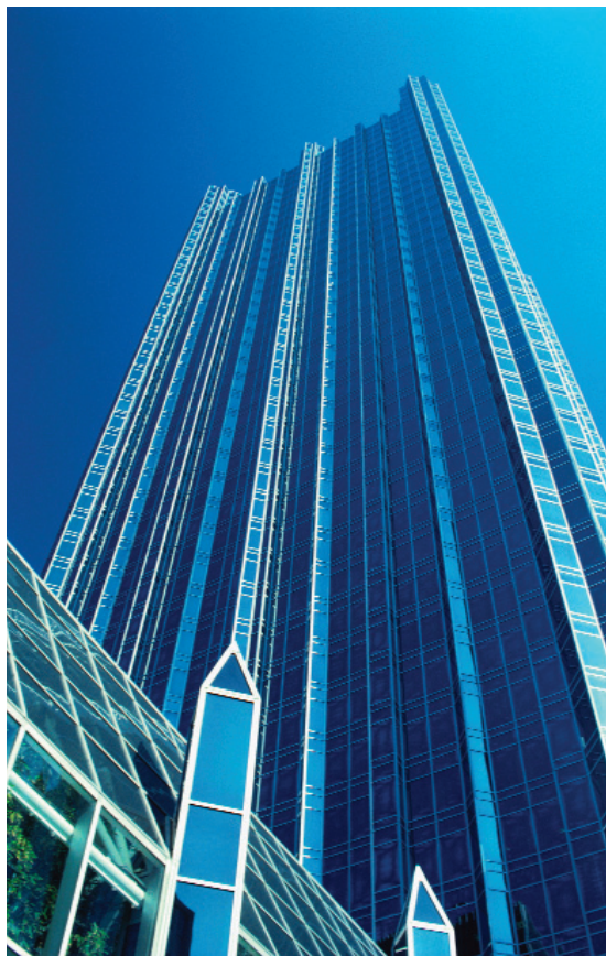
Standards need to be maintained in commercial premises if valuable tenants are to be retained
